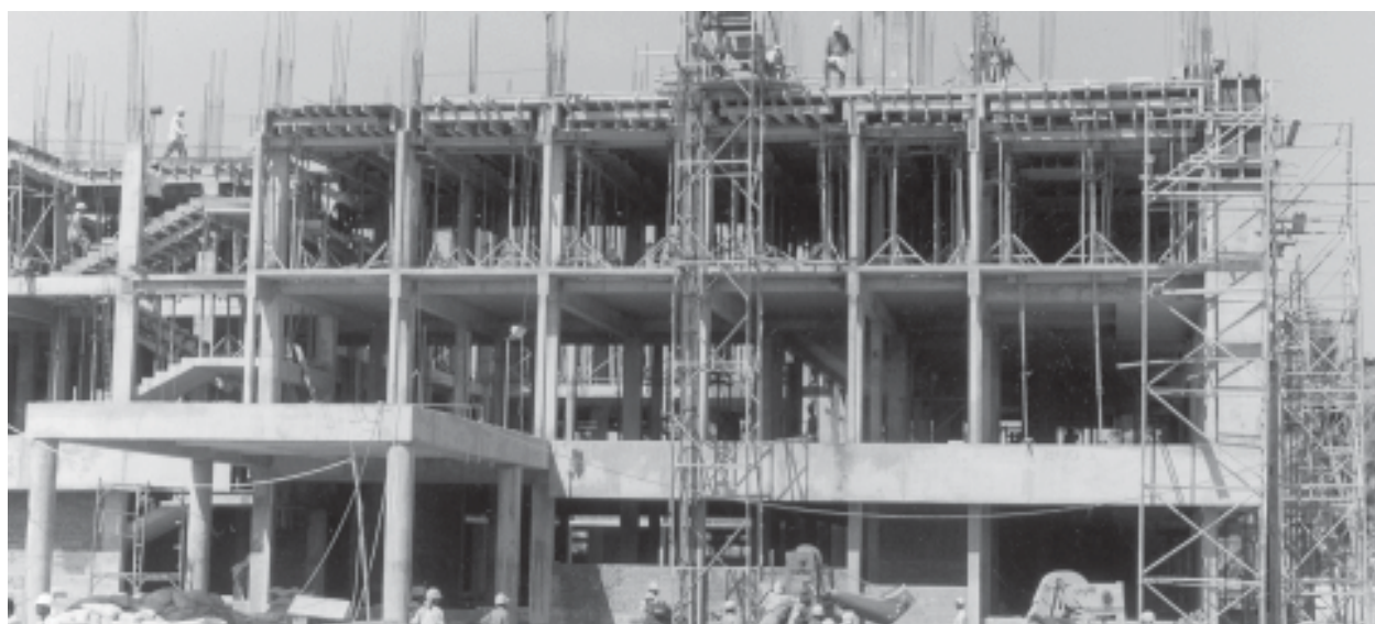
Construction of Aravind-Pondicherry
